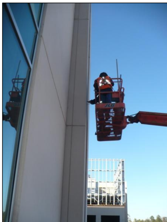
Figure 35 - Performing Probing Sealant Test. Courtesy SGH
