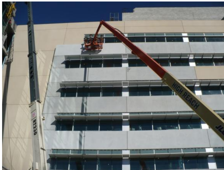
Figure 3 - Installation of Sun shading Device. Courtesy SGH.
